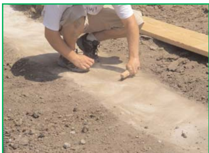
CMUs were adhered directly to a floating foundation using Mason Bond™ from ITW TACC.
