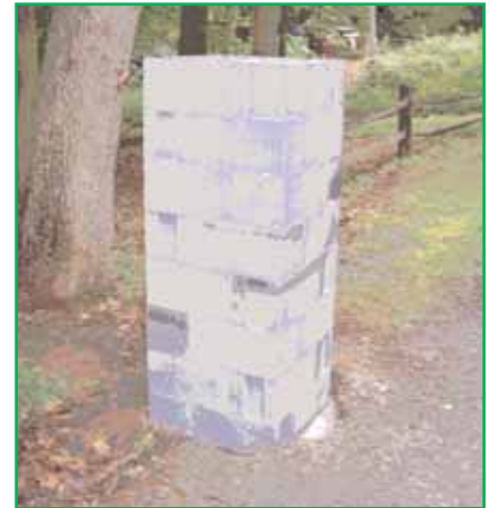
A finished pillar. Louis Seaman completed two pillars in just 57 minutes!
