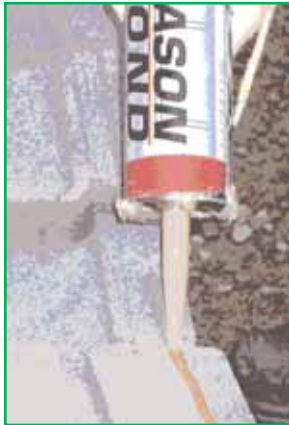
Mason Bond™ applied to vertical surface of the masonry block before it is set in place.
