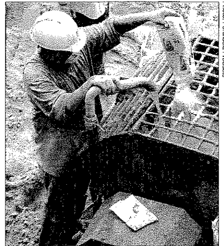
Easy Spred is added to mortar in 7-pound bags to replace 50 pounds of lime.
